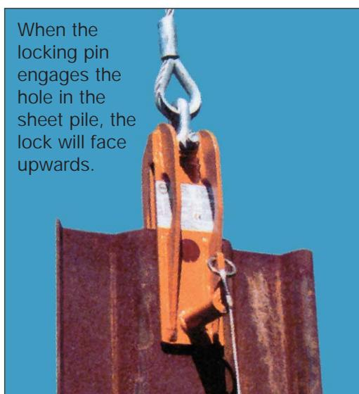
When the locking pin engages the hole in the sheet pile, the lock will face upwards.
