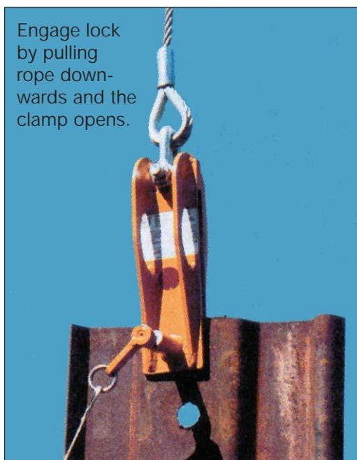
Engage lock by pulling rope downwards and the clamp opens.
